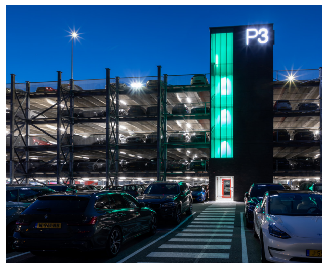
Car park P3, Eindhoven Airport
